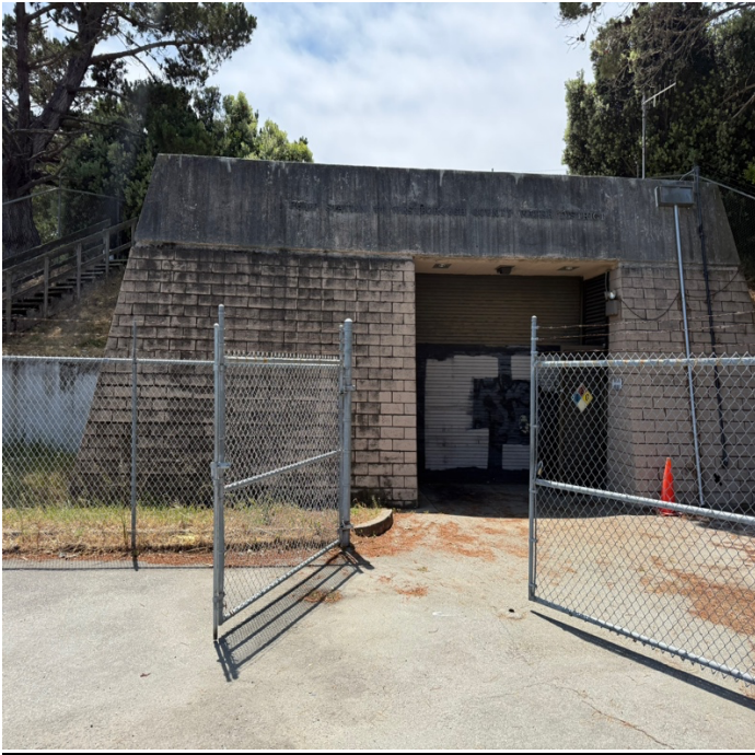
Photo 5: Inspection of Roundtree Lift Station (view 1).
