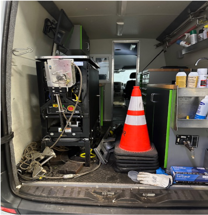
Photo 5: Inspection of Daly City CCTV equipment (view 1).
