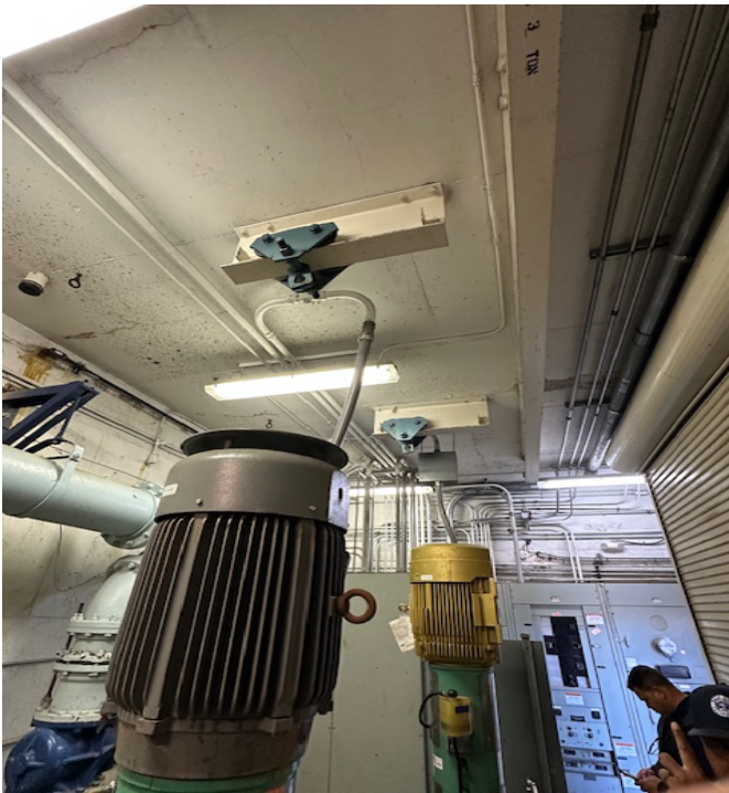
Photo 7: Inspection of Roundtree Lift Station (view 3).
