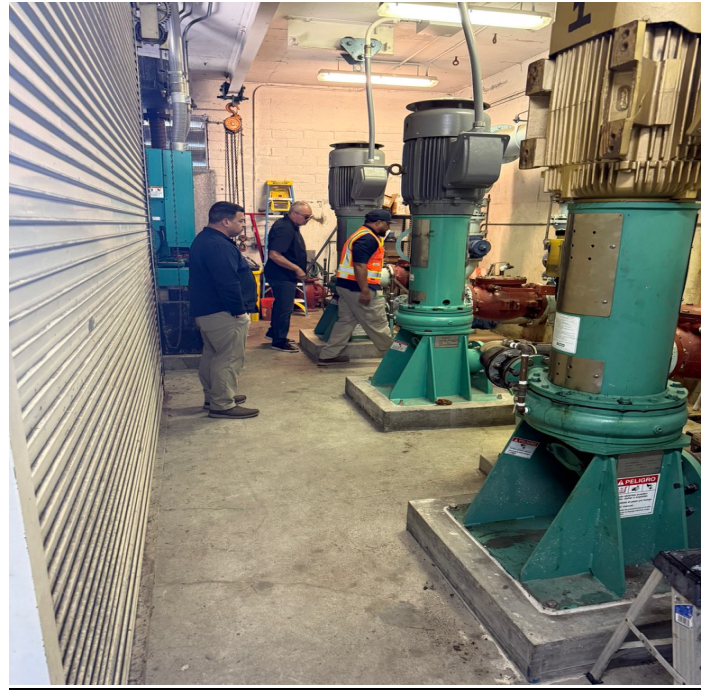
Photo 6: Inspection of Roundtree Lift Station (view 2).
