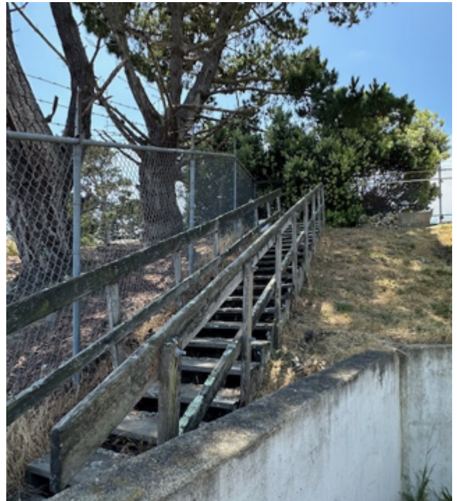
Photo 8: Inspection of Roundtree Lift Station (view 3).
